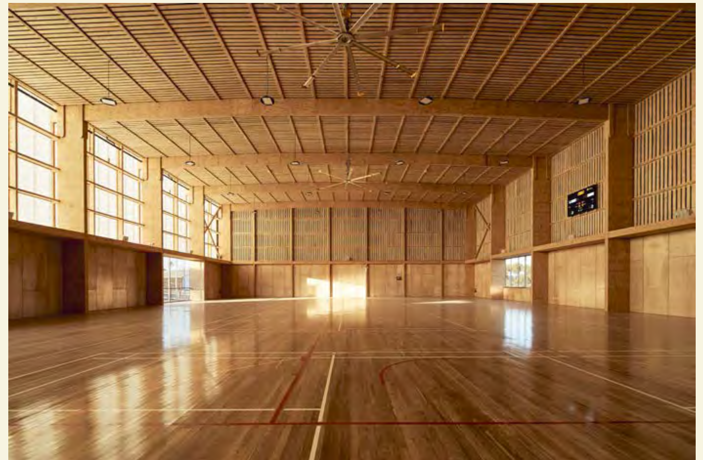
PINGELLY RECREATION AND CULTURAL CENTRE / IREDALE PEDERSON HOOK AND ADVANCED TIMBER CONCEPTS STUDIO PHOTOGRAPHY: PETER BENNETTS
